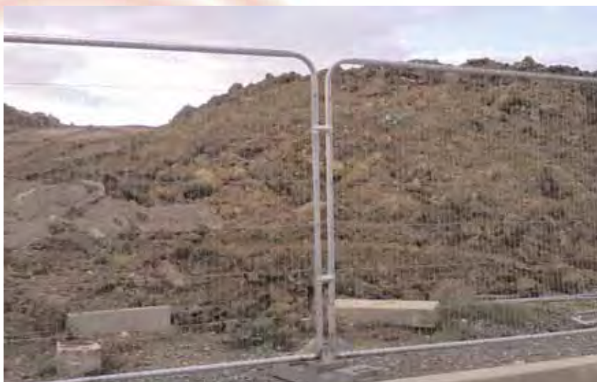
Soil stored on a construction site.
