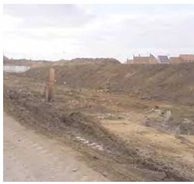
Soil compacted during a construction project.
